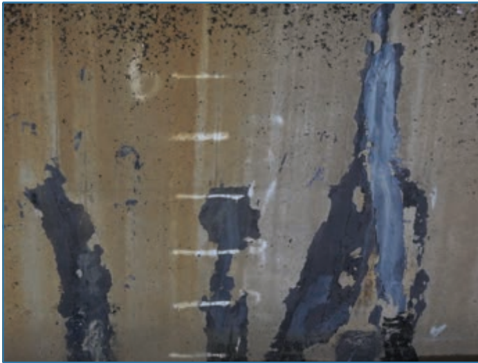
Tar Crack Filling on Spillway
