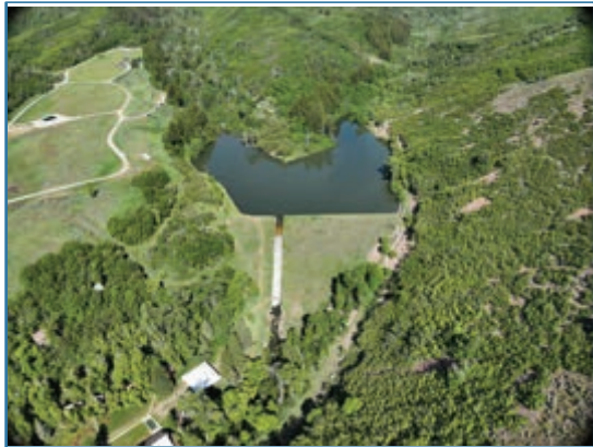
Aerial View of Dam
