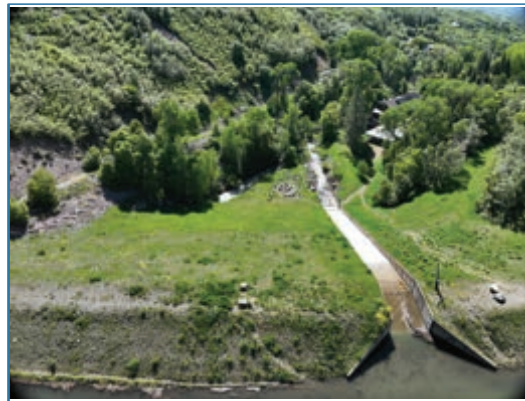
Top of Spillway
