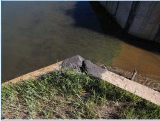
Corner of Spillway
